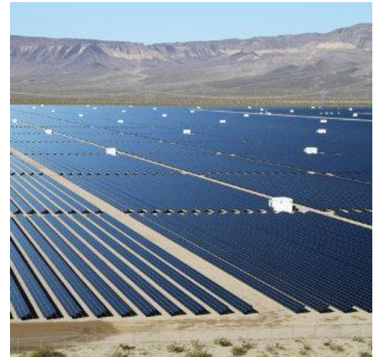
Copper Mountain Solar
